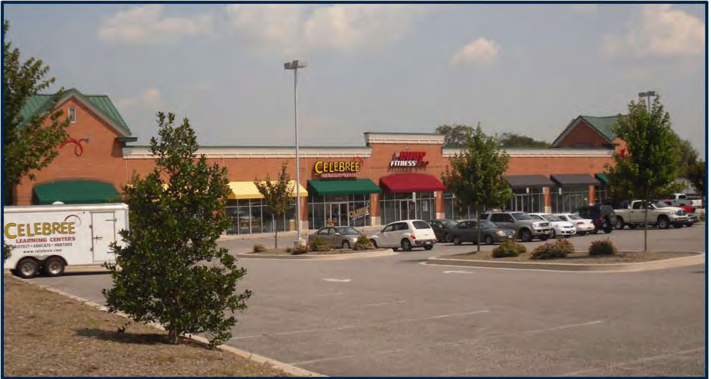
lot 4 building photo
