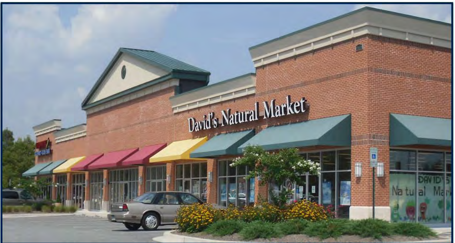
lot 1 building photo
