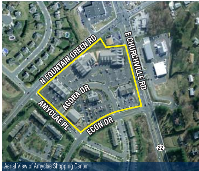
View of 1204 Agora Drive
