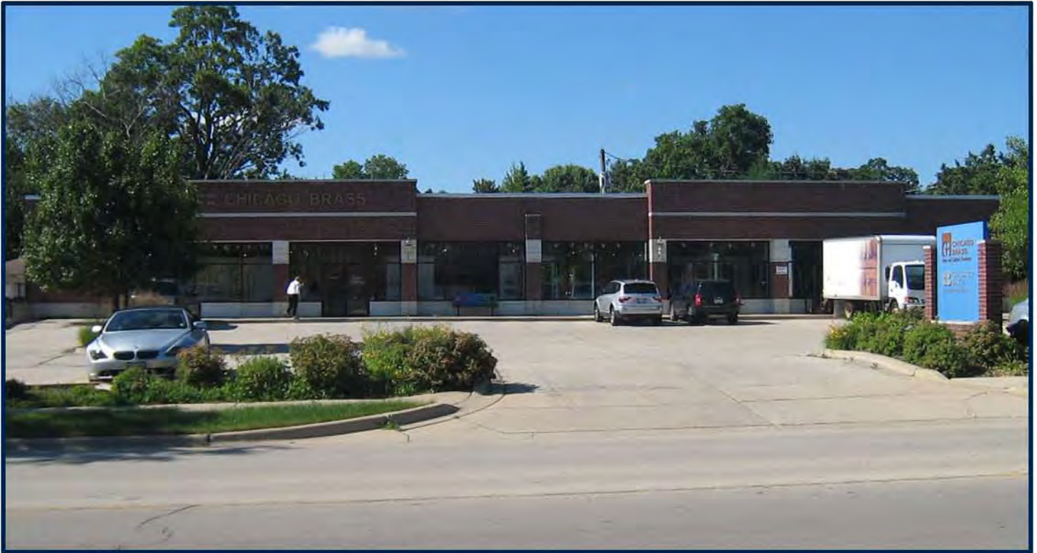
view of building from across Prairie Avenue
