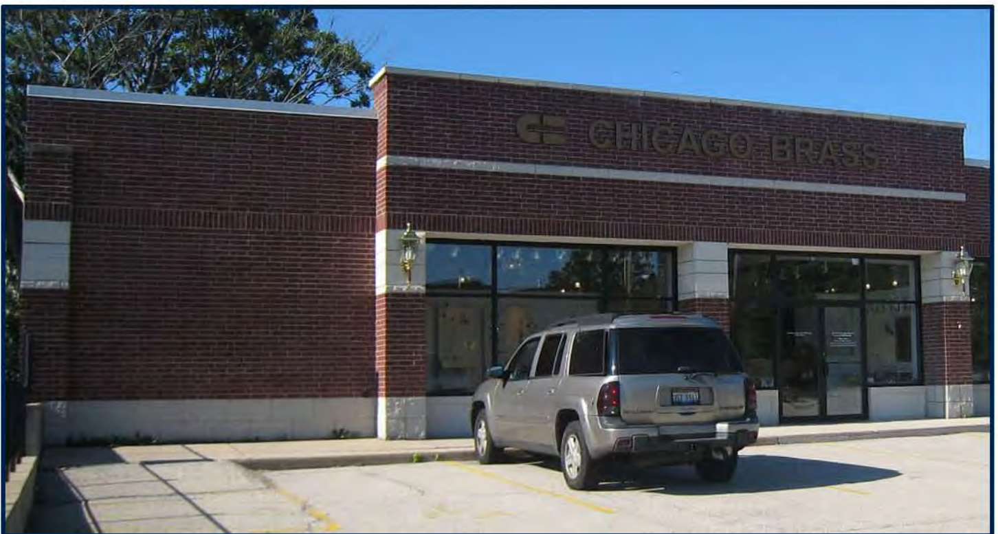
detail of building facade
