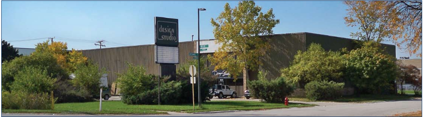
Photo of Building from Busse Road
