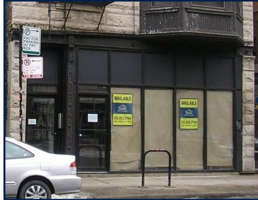
Lincoln Avenue entrance
